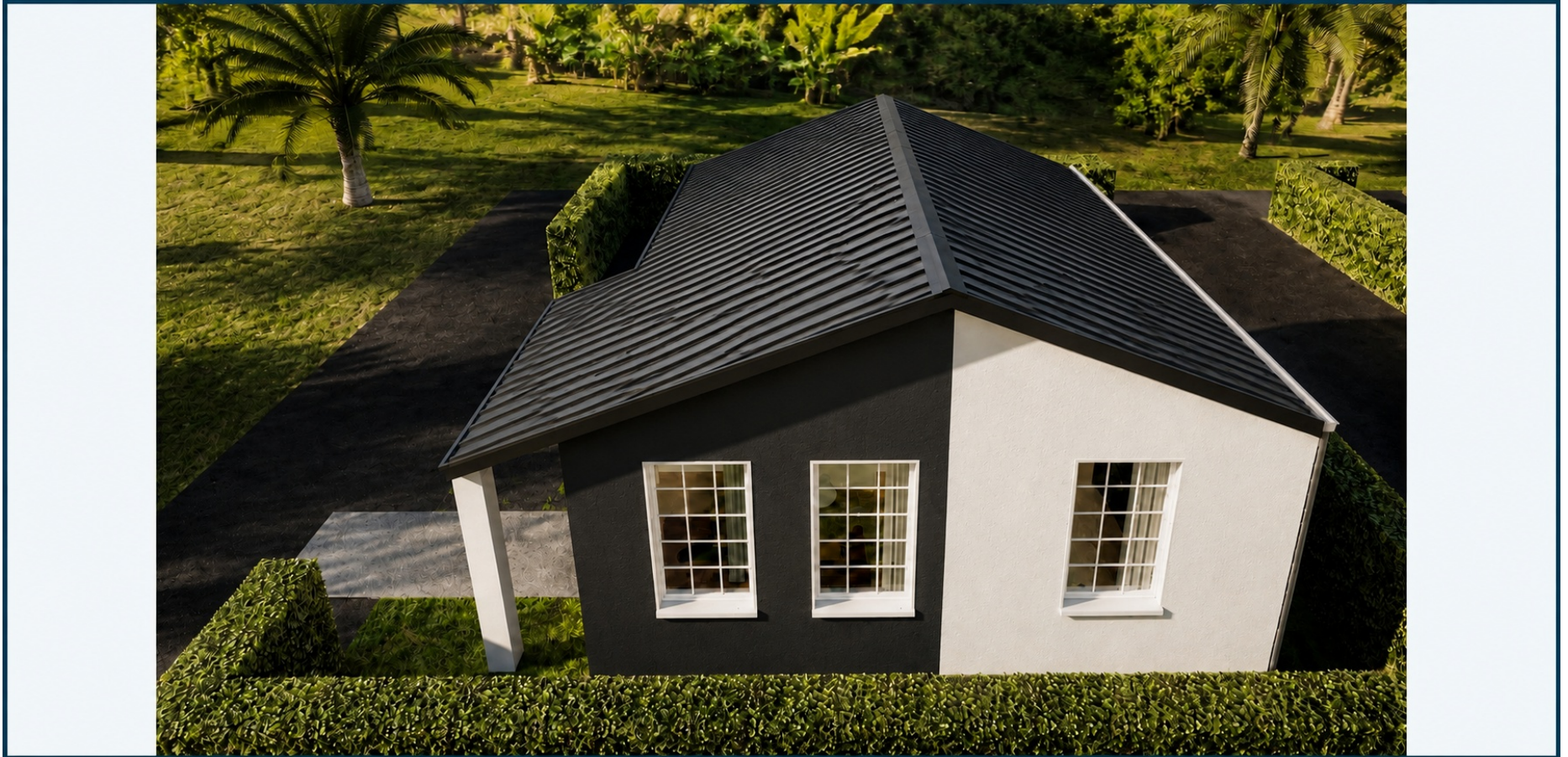
Side-window composition with dark corrugated zinc-sheet roofing and ridge flashing
