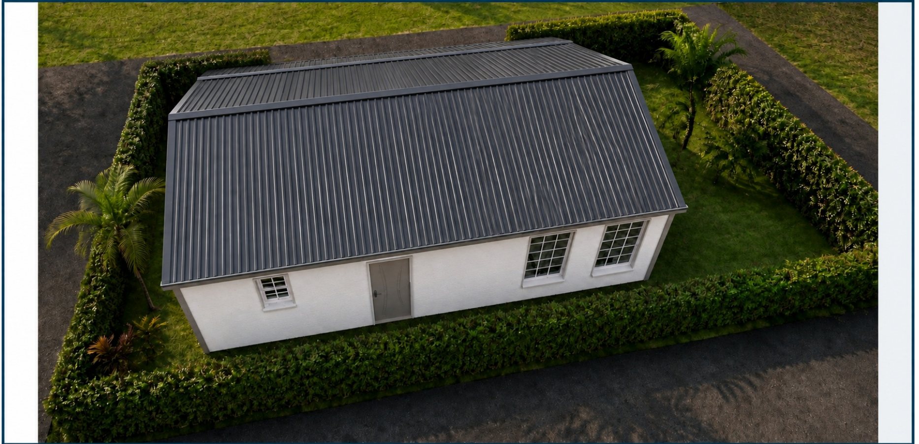
Rear access and service-side windows beneath the corrugated zinc-sheet roof
