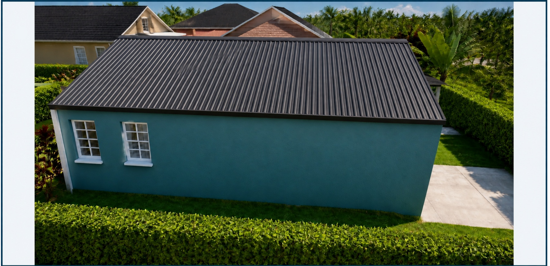
Long side elevation with teal exterior finish, corrugated zinc roofing and balanced windows.
