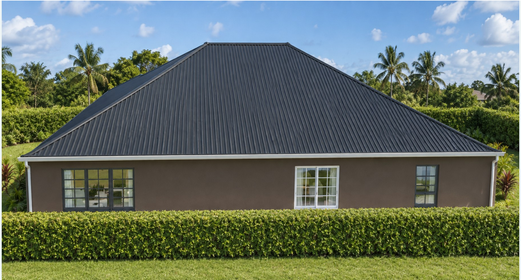
Rear architectural view with the original opening arrangement, zinc-sheet roof and landscaped boundary.
