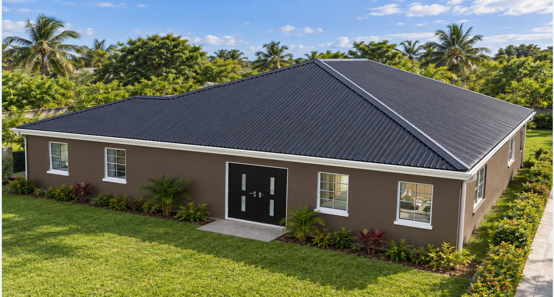
Elevated side and rear entrance view showing the compound zinc-sheet hip roof and secondary access.
